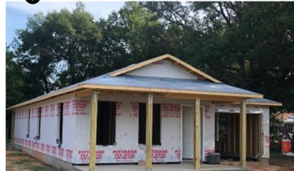
UNDER CONSTRUCTION 226 Milton Road
