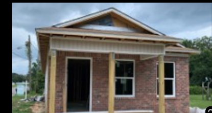
Under Construction 2424 N. Guillemard Street
