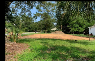
UNDER CONSTRUCTION 920 North L Street
