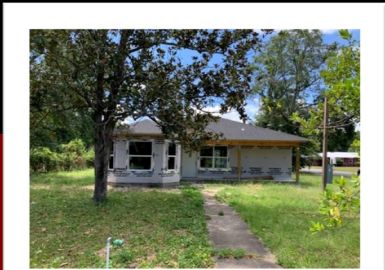
UNDER CONSTRUCTION 1827 North A Street
